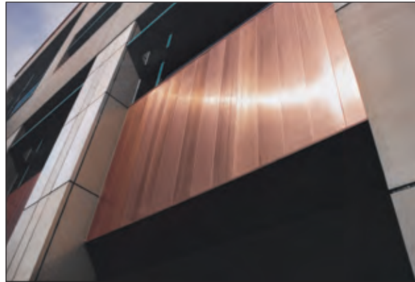
Figure VI-11. The Anchor Center office building in Scottsdale, Arizona, chose to boast its location in the Copper State by preserving the natural color of freshly milled copper sheet with a clear coating. Due to sun and heat, the finish requires reapplication every few years to maintain its pristine look.
