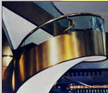
Figure IV-2. Copper alloys installed on this staircase at the European American Bank, New York, New York are examples of simple bending. The handrail is a solid extrusion of architectural bronze, C38500; stringer cladding is Muntz metal, C28000.
