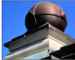
Figure IV-10. Copper globes, fabricated from spun and brake-formed components, adorn four towers at the corners of the Ellis Island Immigration Museum in New York Harbor, New York, New York.
