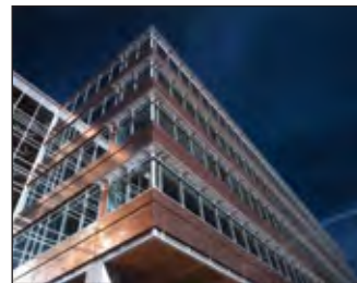
Figure IV-11. Copper laminate panels, from ALPOLIC, wrapping the Ceridian Corporation Headquarters in Minneapolis, Minnesota, will naturally weather in harmony with its surroundings.
