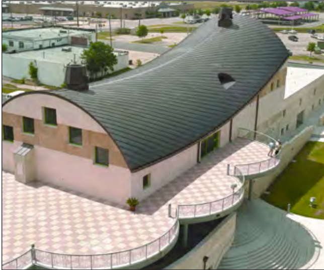
Figure IV-4. The long, diagonal panels gracing the saddle-roof of the San Angelo Museum, San Angelo, Texas, provide a distinctive perspective of the structure from all angles; HHPA, architect.
