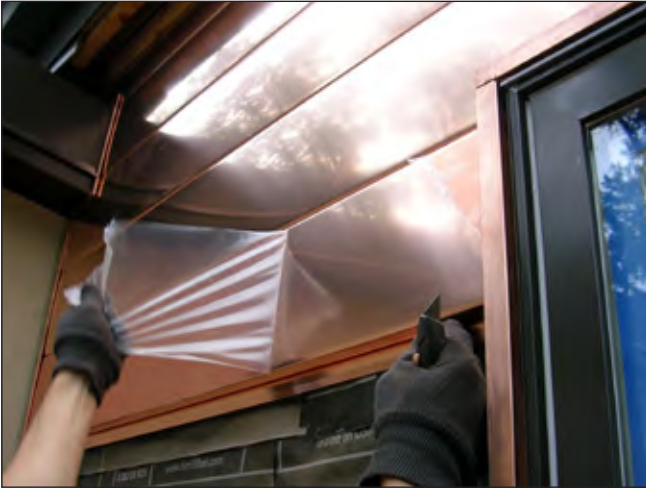
Figure V-9. Careful handling, use of gloves and even protective films can potentially protect copper alloy surfaces and may prevent marring or discoloration from skin oils.
