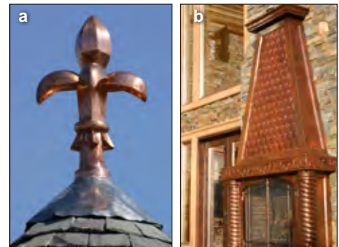
Figure II-2. Extremely malleable, soft temper copper is the ideal medium for this finial ( a ) and hand hammered repousse fireplace mantle with spiral columns ( b ).
