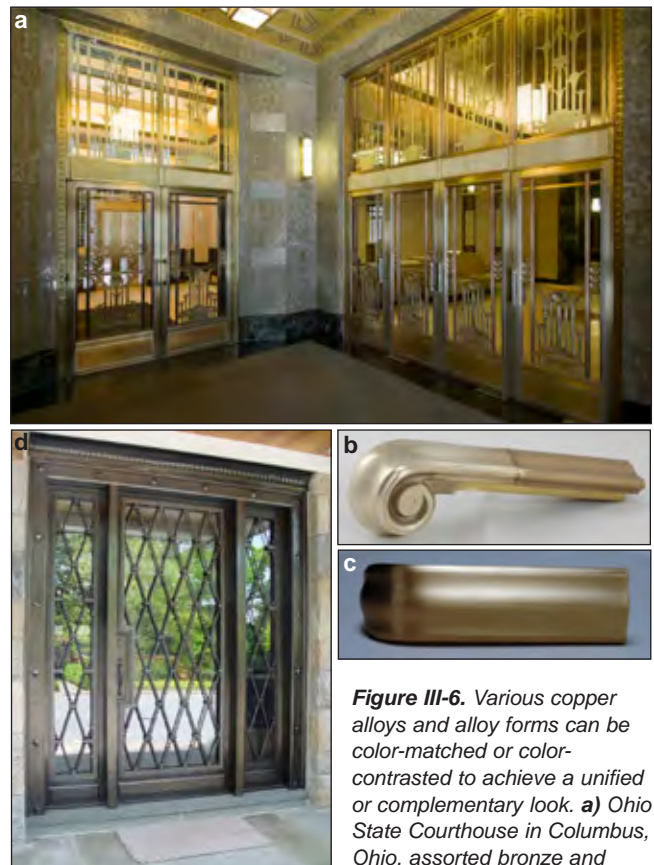
Figure III-6. Various copper alloys and alloy forms can be color-matched or color-contrasted to achieve a unified or complementary look. a) Ohio State Courthouse in Columbus, Ohio, assorted bronze and nickel silver extrusions by Mac Metals. b, c) Extruded architectural bronze (C38500) cast cap brazed to a cast ounce metal (C83600) volute and finished to a seamless appearance, R & B Wagner, Inc. d) Although this door and sidelight set are manufactured from three copper alloys of very different color tones, Wiemann Metalcraft used chemical weathering techniques for a perfect color match.
