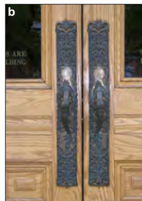
Figure II-4. a) This cast and fabricated bronze balcony railing for an Indiana residence features no visible welds or fasteners. The component pieces were press-fit together using roll pins. Water-jet cutting speeded fabrication of many design elements. The finish is a satin grain (180-220 grit) with a clear lacquer. b) Cast bronze door hardware at Salt Lake City Hall, Utah. c) Custom, hand-forged, bronze handrail.
