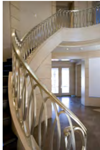
Figure II-7. Fabricated by DeAngelis Ironwork Inc., South Easton, Massachusetts, from all nickel silver components from Julius Blum. The top rail is a molded cap. The interlocking oval segments were formed hot and brazed to one another. Fasteners were concealed by brazing in matching nickel silver plugs. All components received a satin brush finish.
