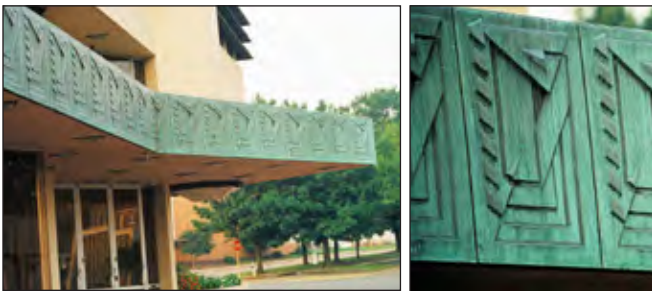
Figure IV-8. Decorative panels on the Frank Lloyd Wright-designed Price Tower in the prairie town of Bartlesville, Oklahoma, demonstrate one of the effects possible from stamping. The vertical copper panels would not have weathered blue-green in this climate, but Wright loved the color and had the panels chemically patinated prior to installation.
