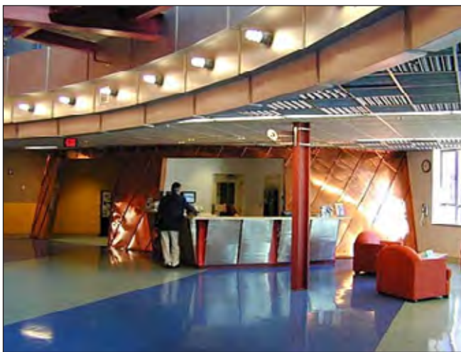
Figure IV-13. Seams between individual sheet copper panels create a decorative pattern in the vestibule of Central Connecticut State University's Student Center in New Britain, Connecticut.
