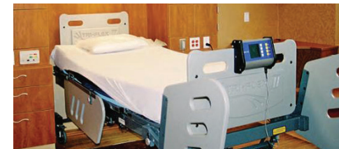
A Carson Tahoe Medical Campus hospital bed outfitted with Category 6+ Cabling. Photo Credit: Superior Essex
