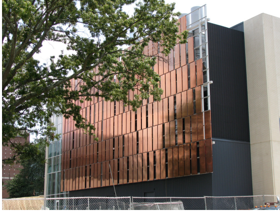
Photo taken during construction by copper panel installer Harmon Inc.
