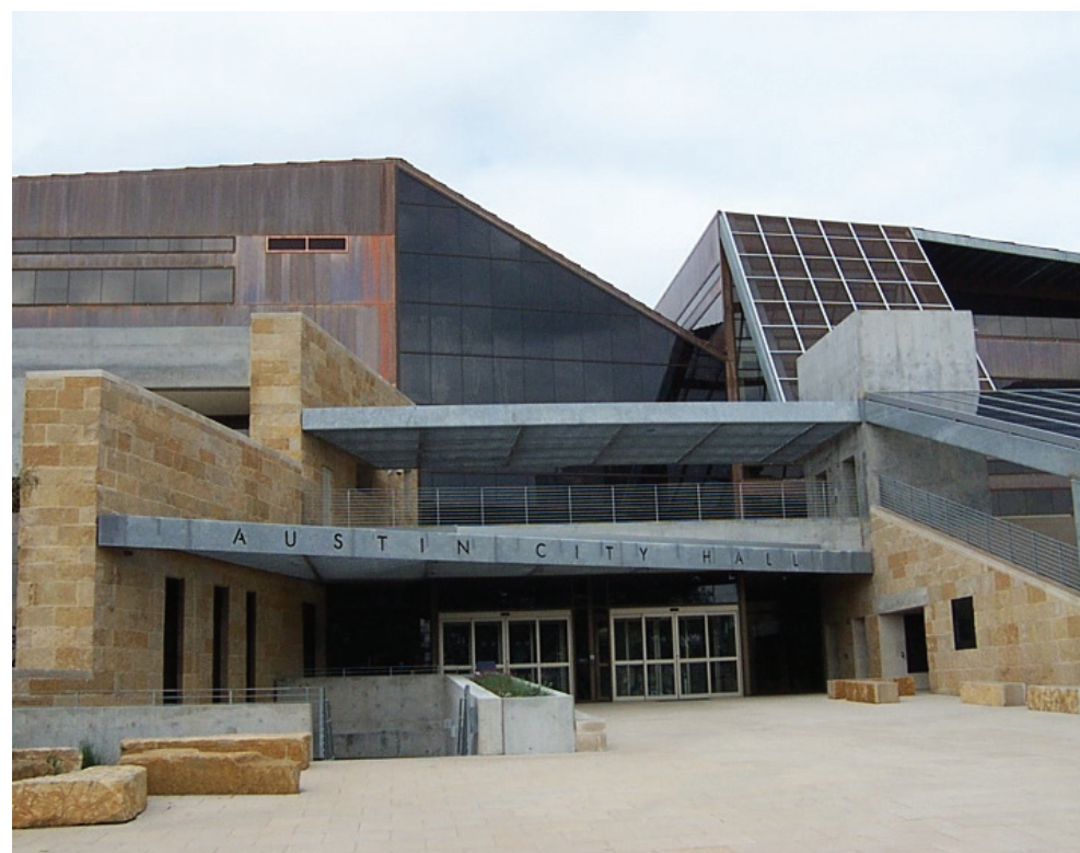
Exterior and interior uses of copper helped Austin City Hall earn USGBC's Gold LEED certification.
