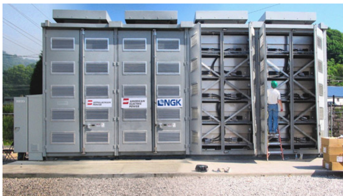
Figure C-3. Altairnano 1 MW/250 kWh Lithium Titanate Battery Trailer and NGK NaS Battery Enclosure
