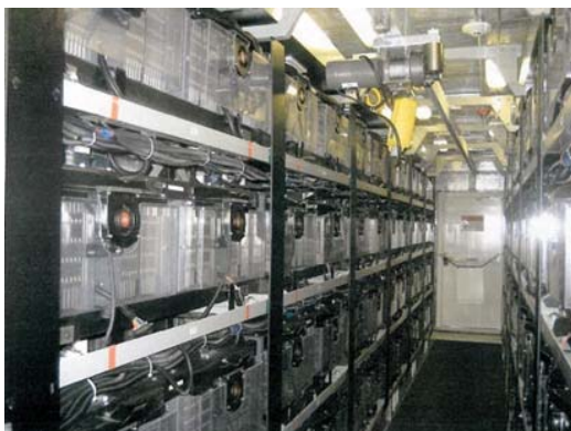
Figure C-3. Altairnano 1 MW/250 kWh Lithium Titanate Battery Trailer and NGK NaS Battery Enclosure
