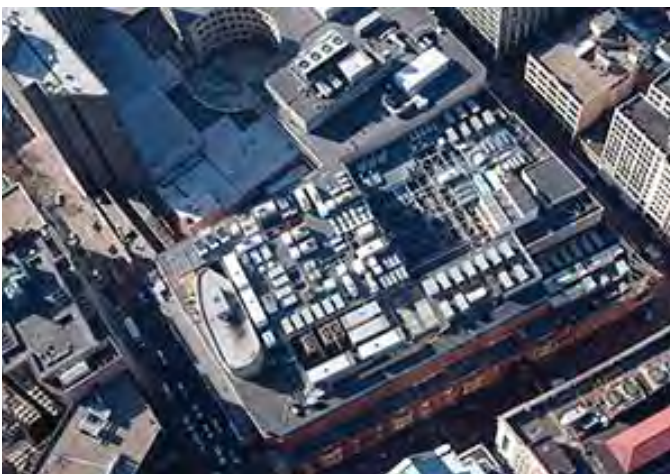
Figure 2. More than 30 generators and HVAC equipment nearly blanket the building's 2½-acre, multitiered roof. A total of 30 MW of emergency power plus more than 10 MW of rotary and battery UPS power ensure seamless transfer. Future build-out to 40 MW of generation will accommodate growing electrical loads.
